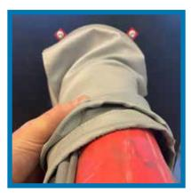
The fireproof wrap should be rotated counterclockwise around the cables to create a smokeproof installation. The more cables that are pulled through the penetration, the closer the cable tie is to the bulkhead. The protrusion of the wrap on the cable varies between 100-300mm depending on the amount of cable in the penetration.
