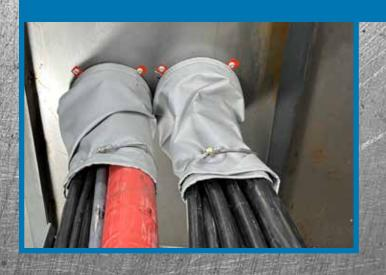
Easy Transit is approved for high cable quantity demand through side by side installation in both deck and bulkhead (2 x Ø160mm). This makes Easy Transit very useful for all above waterline applications.
