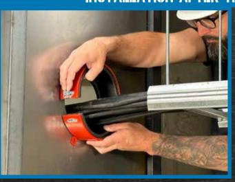
The ability to carry out installation work after the cables have been pulled enhances efficiency, reduces potential disruptions, and streamlines the entire installation process. This method offers flexibility and convenience, while maintaining the integrity of the cable infrastructure.
