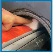
The Blanket insulation that are left over after sealing the voids between the cables and the wrap, can be saved for future retrofit needs. Insert the remaining piece of Blanket into the Easy Transit wrap from the exposed backside.
