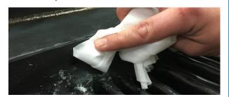
Before any repair, grease, oil and soap must be removed from the area to be repaired.
