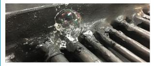
Inspect opposite sides of the sleeve for signs of leakage by using a leak indicating solution (soap water).
