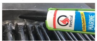
Repair any leakage detected using Marine Flex Silicone. After after curing, repete from step 2,1.
