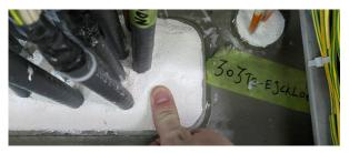
After sealant has cured, use a non-sharp object or your thumb and press into the sealant to detect if at any point the object/thumb penetrates the sealant which would indicate the thickness of sealant is not achieved. Alternatively, a knife can be used to carefully cut away a small piece of the sealant (i.e.20x20mm or 0,8") and then verify the min thickness that is described in the PDA. Reseal with Marine Flex Sealant.
